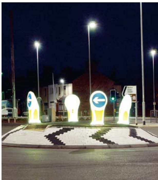
This roundabout has four rotationally molded Simmonsins bollards to help night drivers safely reach their destination.
